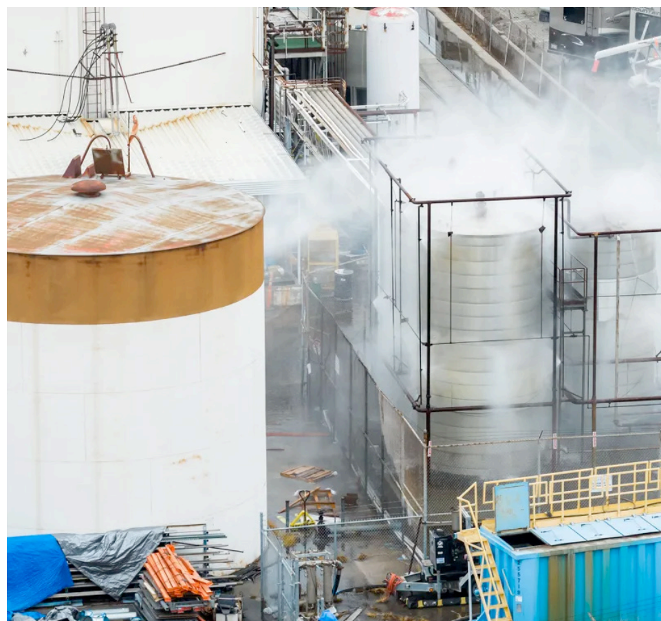
Water is sprayed on a damaged tank at GKN Aerospace in Garden Grove, on May 24, 2026, after the tank containing a chemical used to make plastic parts overheated Thursday. Photo by Ethan Swope, AP Photo
